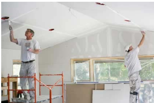
Photo 3. Substituting low-VOC paint reduces odor in occupied space.
