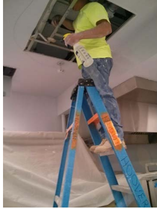
Photo 6. Cleaning construction dust above the ceiling.
